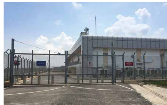
➔ New ancillary buildings, like this airfield lighting control centre, were constructed
